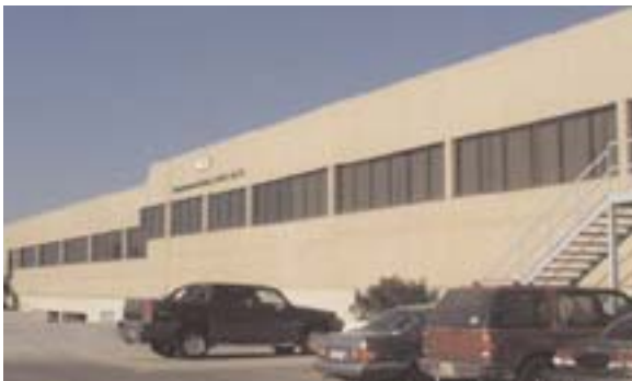
BCLM production facility
